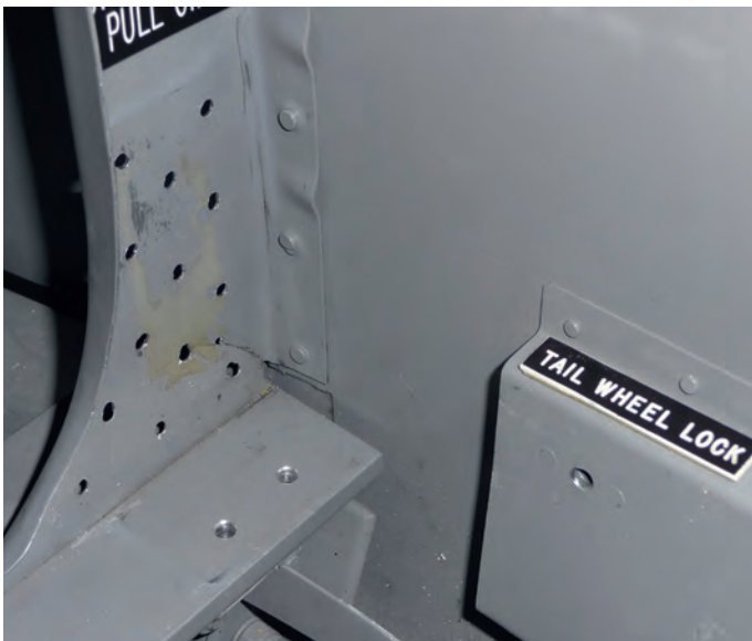
When Roy drilled out the rivets he was aghast to find that the frame had cracked through; note the stop drill at the end of the crack – clearly the engineer who did this was rather behind the common sense curve. (Photo: Roy Holder)
